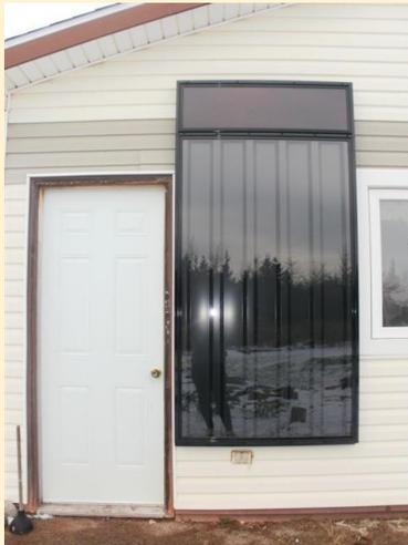
This is the Solarsheat solar heater attached to a south (more or less) facing wall of the cottage.
